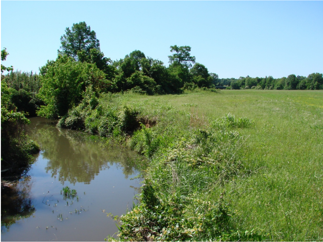
Figure 10. View of eroding stream bank on Little Creek (April 2012).
